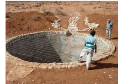
Stone masonry round berked under construction showing wires for roofing materials, Somaliland
