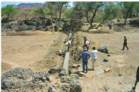
Sub-surface dam under construction VSF (2006). SubSurface Dams : a simple, safe and affordable technology for pastoralists. A manual on SubSurface Dams construction based on an experience of Vétérinaires Sans Frontières in Turkana District (Kenva). September 2006.
