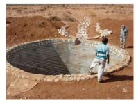
Stone masonry round berked under construction showing wires for roofing materials, Somaliland Eric Fewster, BushProof / Caritas
