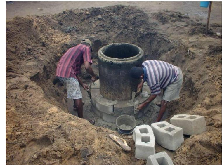
Figure 8: Flood-proofed well, Madagascar – exterior raised headwall under construction
