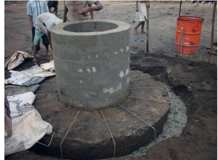
Figure 7: Deeper edges to apron to prevent erosion and undercutting, Madagascar
