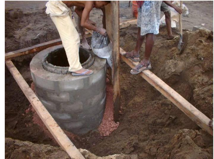
Figure 9: Flood-proofed well, Madagascar – clay grout being added
