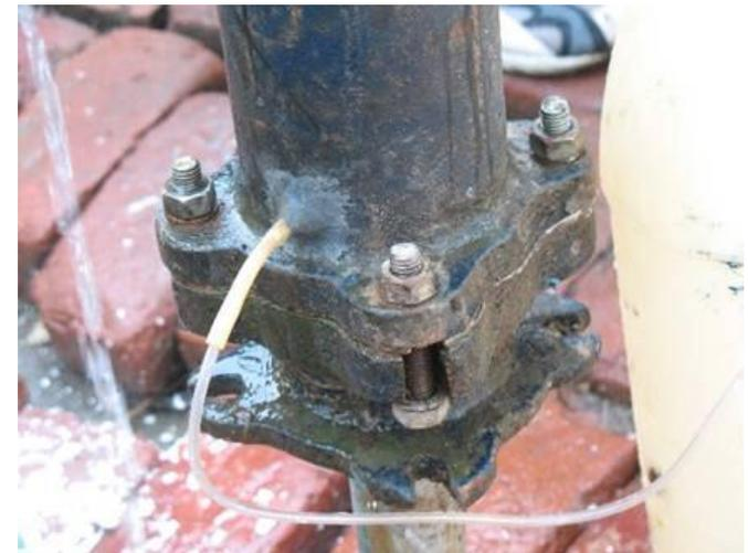
Figure 16: Online chlorination of suction handpump
