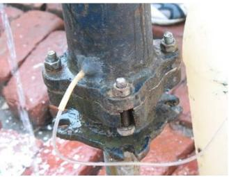
Figure 16: Online chlorination of suction handpump Rasal, P. (2008) Online chlorination of hand pumps, Supaul District, Bihar
