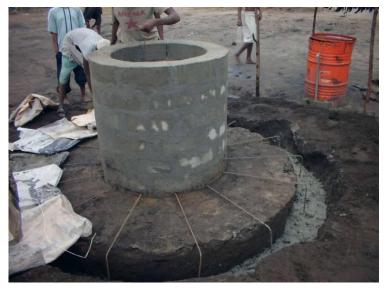
Figure 7: Deeper edges to apron to prevent erosion and undercutting, Madagascar Eric Fewster, Medair
